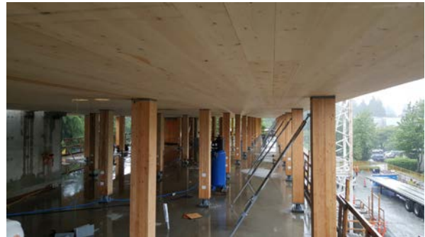
Figure 6. Installed during typical BC weather conditions
