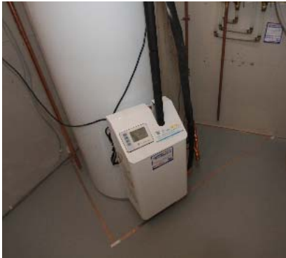
Figure 6. Hot water tank
