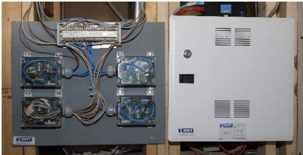
Figure 13. WiDAQs and Building Intelligence Gateway Installed in Utility Room
