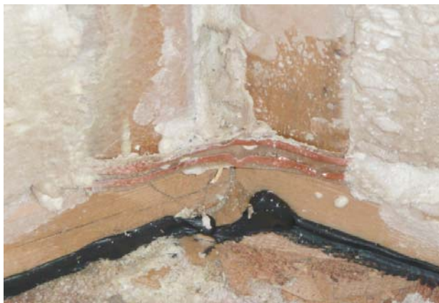
Figure 1. Linear Detection under Icynene Insulation
