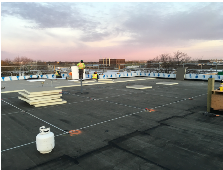
Figure 2. Sensor Grid Installation
