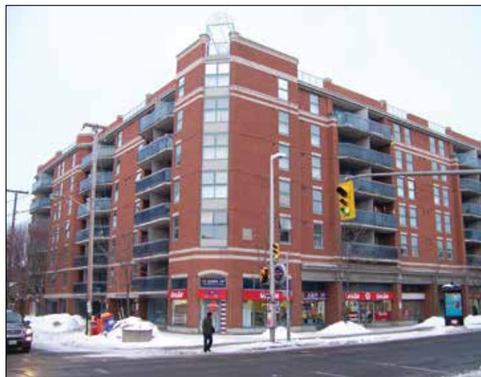
Figure 1 Test building in downtown Ottawa, Ontario.
