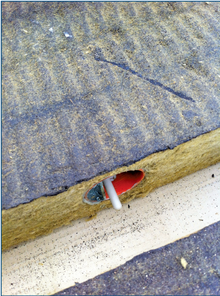
Figure 6 – Displacement sensor mounted in fiberglass tube within insulation core prior to setting of insulation board.
