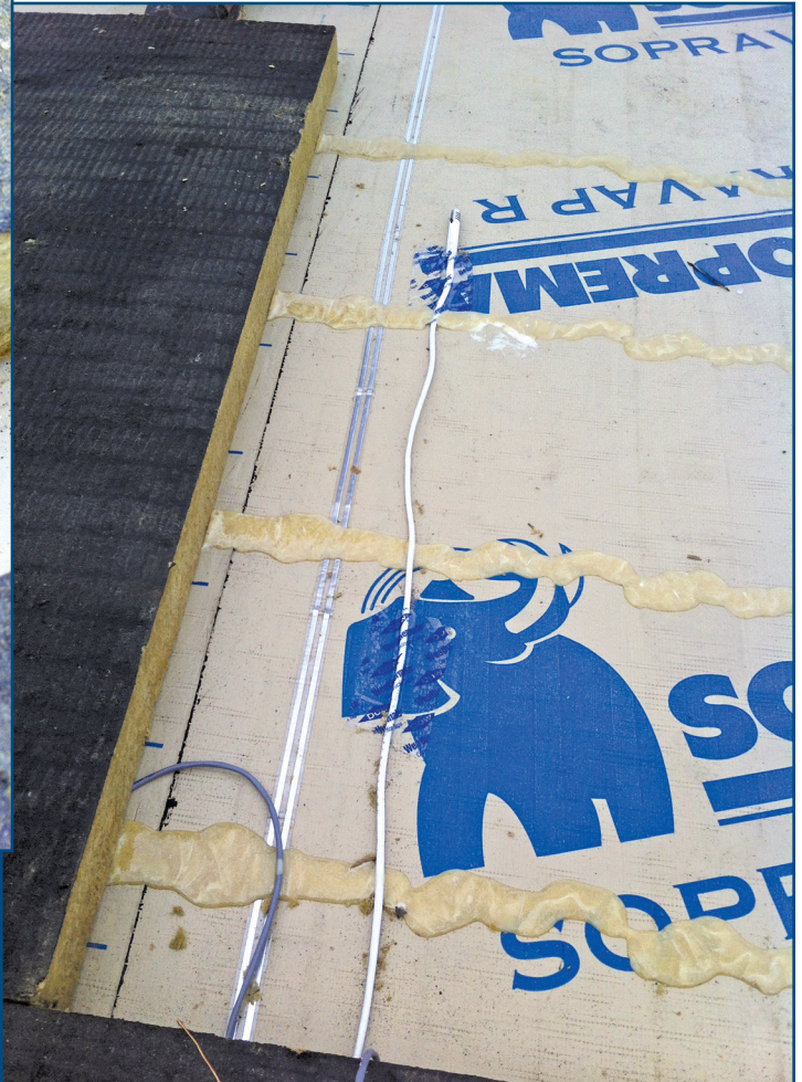
Figure 7 – Moisture detection tape (left) and RH sensor (right) above air/vapour barrier below insulation. Note also the ribbons of adhesive.
