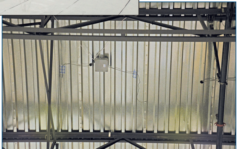
Figure 11 – Interior view of data logger and two interior temperature sensors (metal deck). Deck flutes run in north-south direction.
