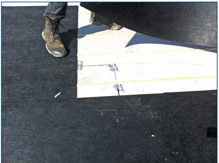
Figure 8 – Top of insulation surface temperature, below asphalt protection board sheet.
