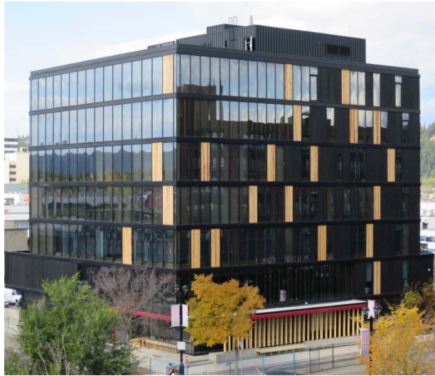
Figure 1 The Wood Innovation and Design Centre in Prince George, British Columbia
