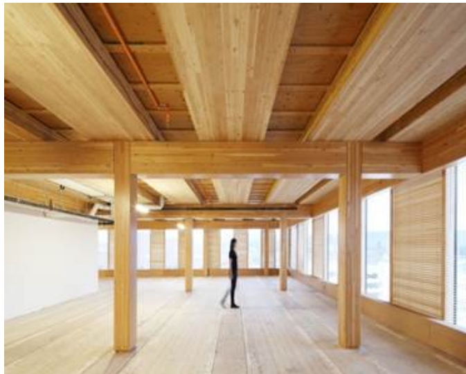
Figure 2 Mass timber roof structure integrated with an interior ventilation cavity between plywood roof sheathing and CLT panels below (Courtesy of Michael Green Architecture)
