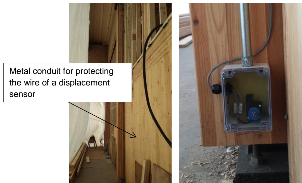
Figure 5 A displacement sensor (its metal conduit in left photo, and a closer image of the sensor box which is adjacent to the column base) at Location 1 for measuring vertical movement of the glulam column
