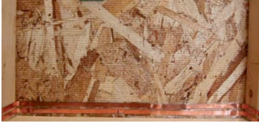
Adhesive tape applied to base zone of building envelope
